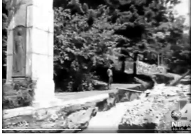
Figure 8 – Ground failures at Memory during the 1983 flood about 600 feet from the proposed Well. Writh, Craig (KUTV News). May 12, 2014. Remembering the flood of '83. KUTV News. At min. 1:35. (url: https://www.abc4.com/wirth/wirth-watching-remembering-the-salt-lake-city-flood-of-83/204262974 ).
